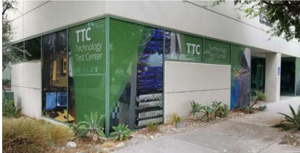
SCE Technology Test Center (TTC)
