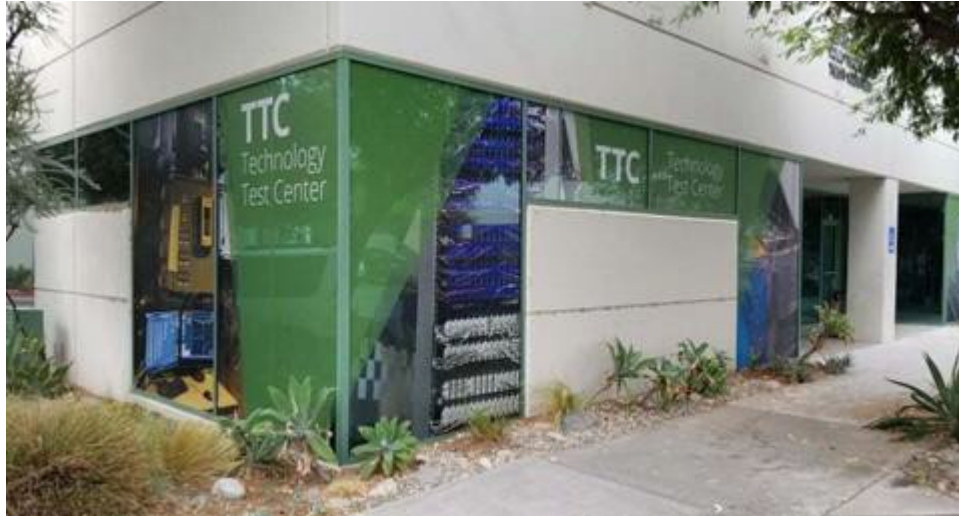
SCE Technology Test Center (TTC)
