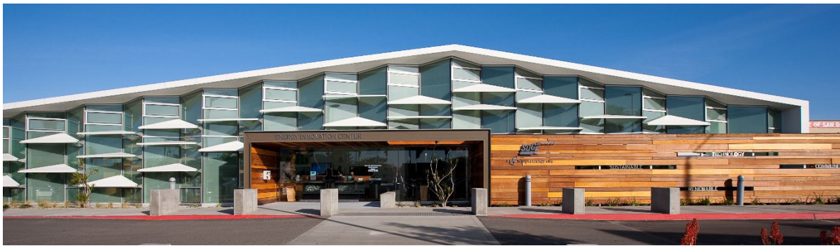
Figure 1. SDG&E Energy Innovation Center – Street Facing View
