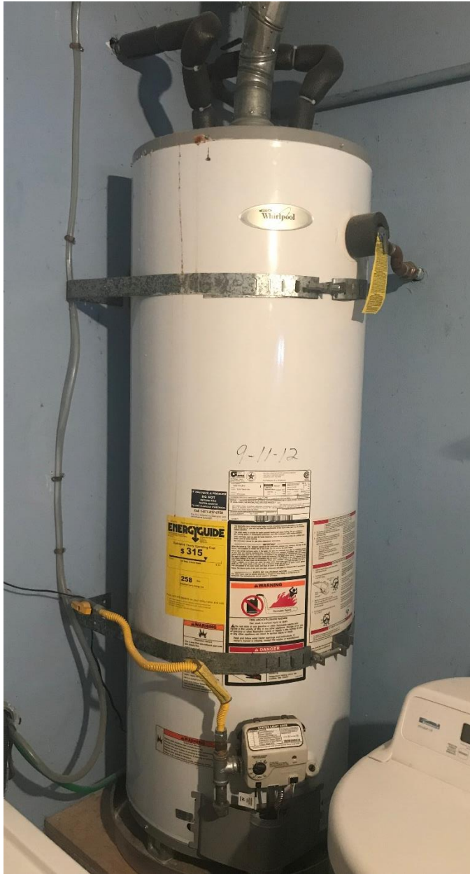
FIGURE 2 – IMAGE OF EXISTING GAS WATER HEATER IN HOME 1
