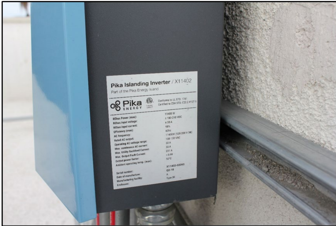
FIGURE 22. INVERTER NAMEPLATE STICKER AND INFORMATION
