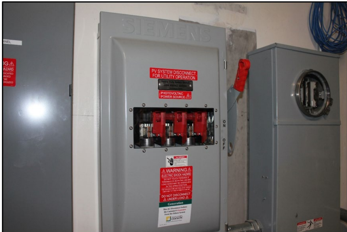
FIGURE 15. UTILITY SOLAR PV DISCONNECT (CENTER) AND JUMPERED METER SOCKET (RIGHT)
