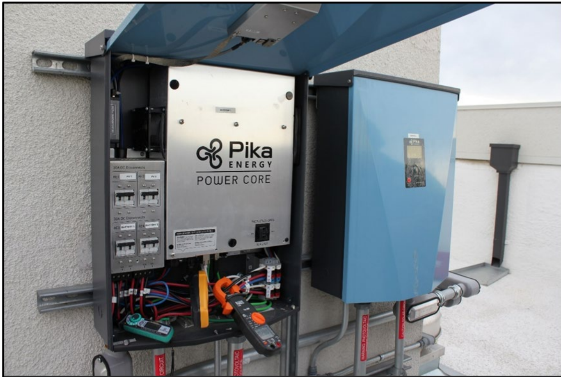
FIGURE 16. INVERTER 1 LID IS OPEN AND INVERTER 2 LID IS CLOSED
