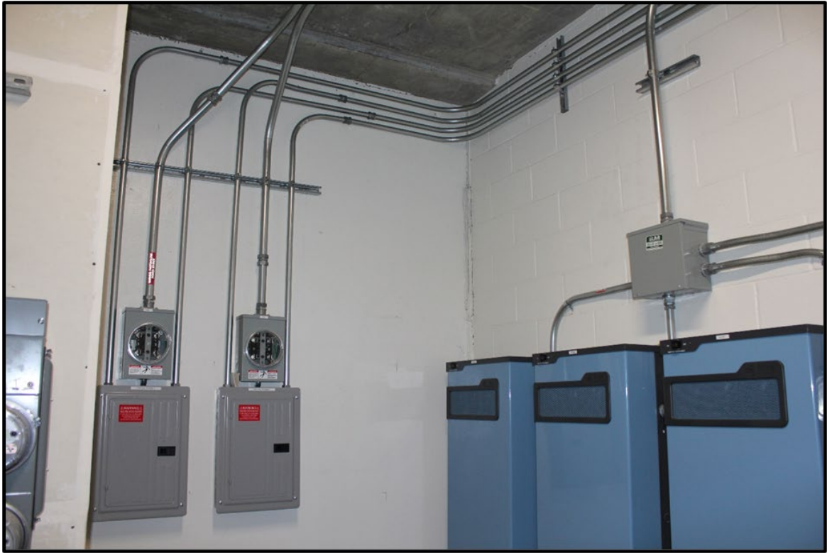
FIGURE 5. ESSENTIAL LOADS BACKUP PANEL (LEFT) AND PIKA HARBOR SMART BATTERIES (RIGHT)
