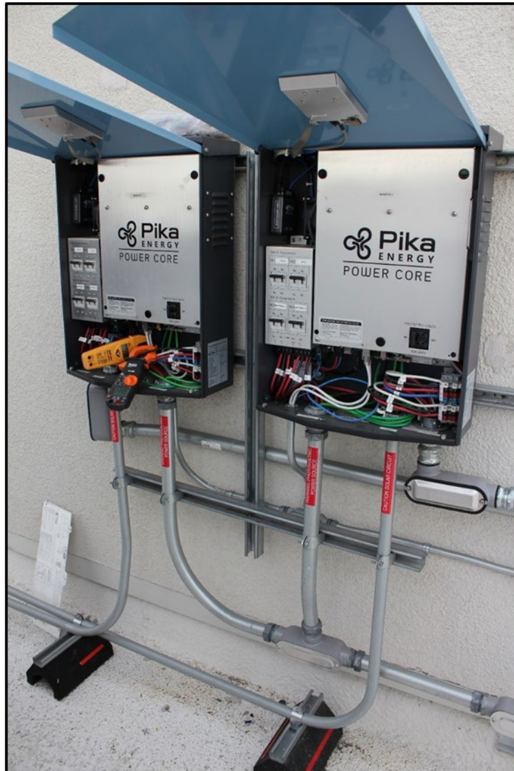
FIGURE 24. BOTH BATTERY INVERTERS WITH OPEN LID COVERS WITH CONDUIT HARDWARE DISPLAYED
