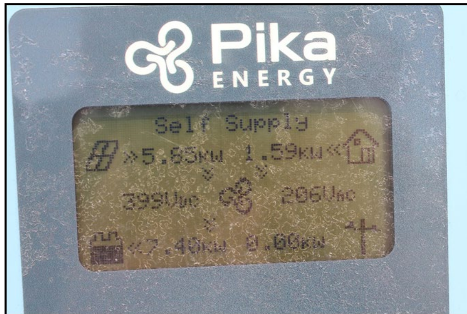
FIGURE 13. INVERTER 2 (INV2) RECEIVING SOLAR PV FROM INVERTER 1 (INV1)
