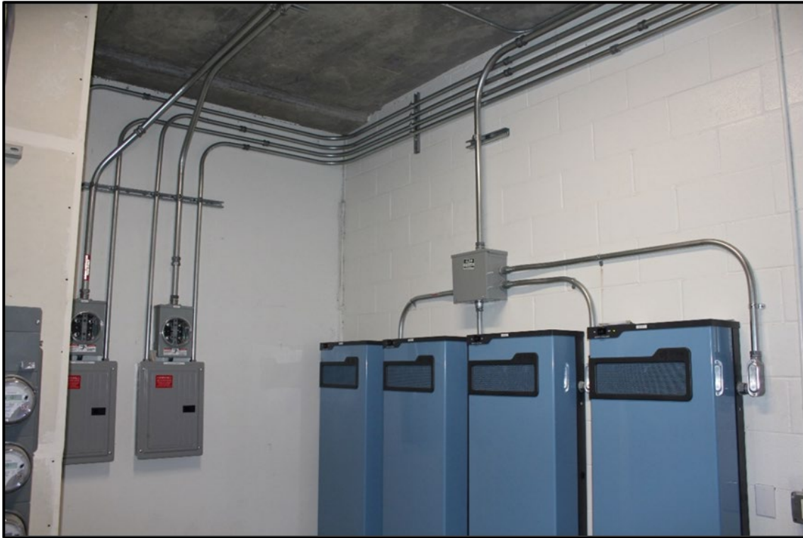
FIGURE 14. ESSENTIAL LOADS BACKUP PANEL (LEFT) AND PIKA HARBOR SMART BATTERIES (RIGHT)
