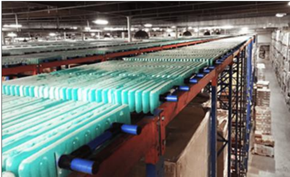
PCM Technology Installed in Warehouse
