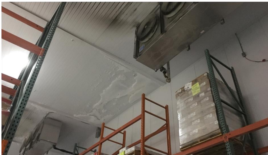
FIGURE 5: FROZEN FOODS WAREHOUSE EVAPORATORS
