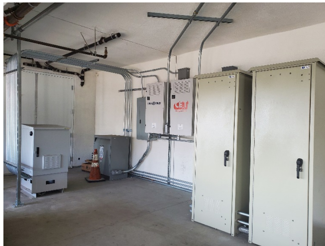
FIGURE 6 - INSTALLED CE+T STABILITI 30C3 INVERTER UNITS (LEFT) AND ENCLOSED ENERGPORT L3060 BATTERIES (RIGHT)
