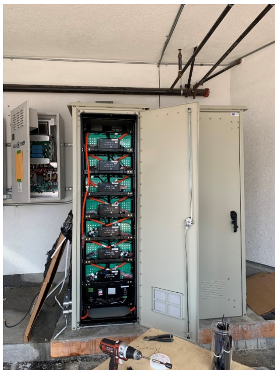
FIGURE 5 - L3060 ENERPORT BATTERY INSTALLATION AT PROJECT SITE
