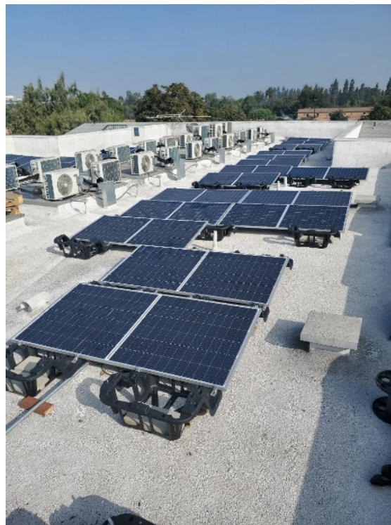
FIGURE 4 - BIFACIAL SOLAR INSTALLATION AT PROJECT SITE
