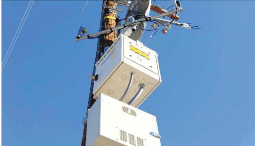
**Figure 4. iDirect Satellite with Wireless On-Ramp Access Point**
