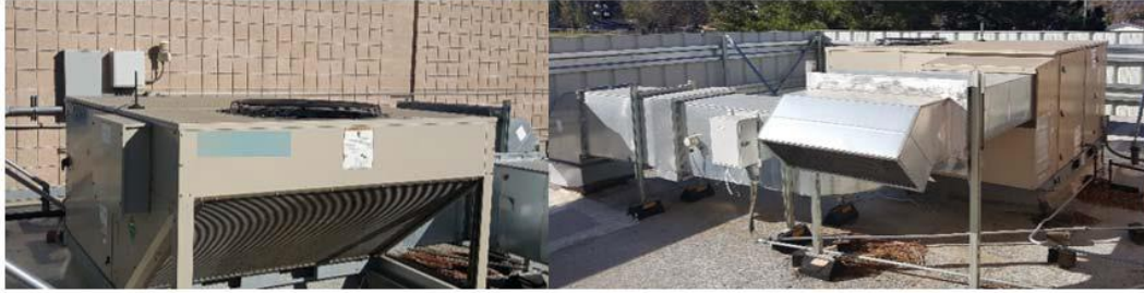
Image: RTU Unit
