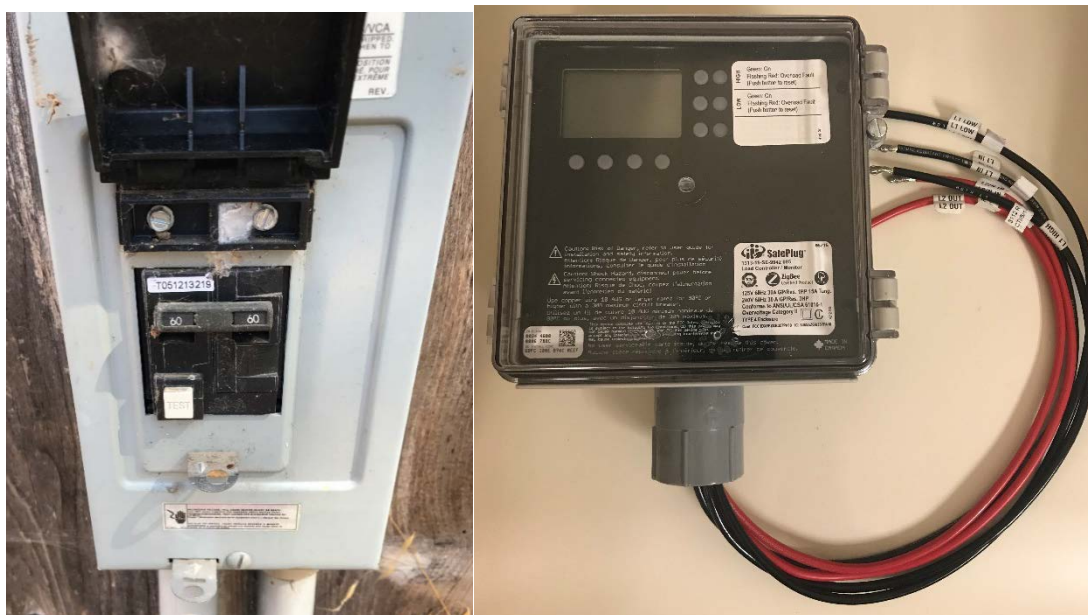
FIGURE 6: (LEFT) BREAKER FOR SPA PUMP AT HOME 2; (RIGHT) HOME 2 DIRECT LOAD CONTROLLER
