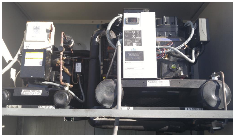
FIGURE 2. – MESS HALL REFRIGERATION UNIT
