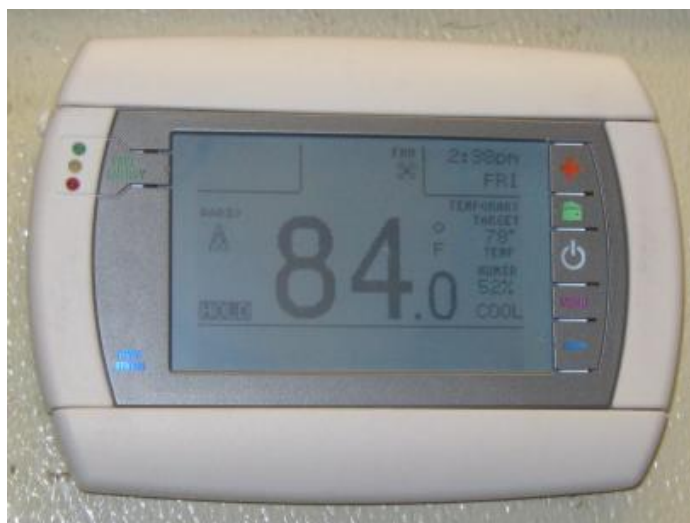
FIGURE 1. PCT MOUNTED ON WALL
