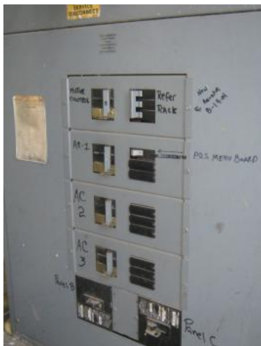
FIGURE 3. AIR CONDITIONER BREAKERS IN ELECTRIC ROOM
