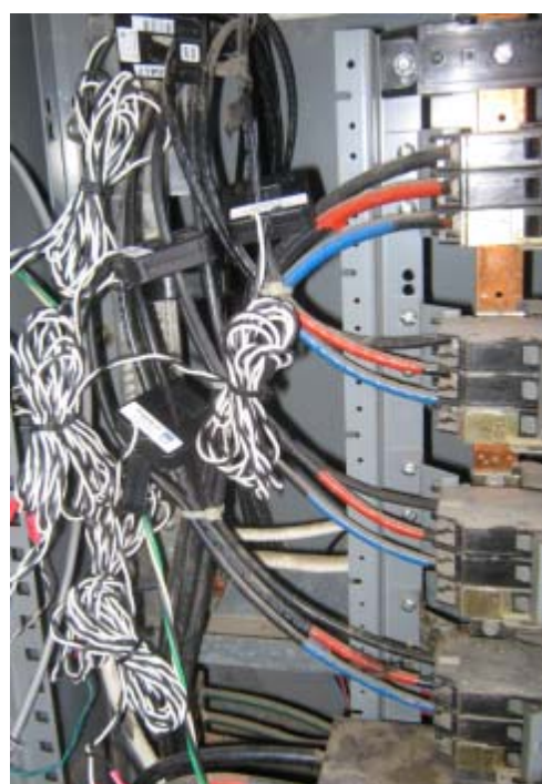
FIGURE 4. CURRENT TRANSDUCERS MOUNTED INSIDE ELECTRIC PANEL
