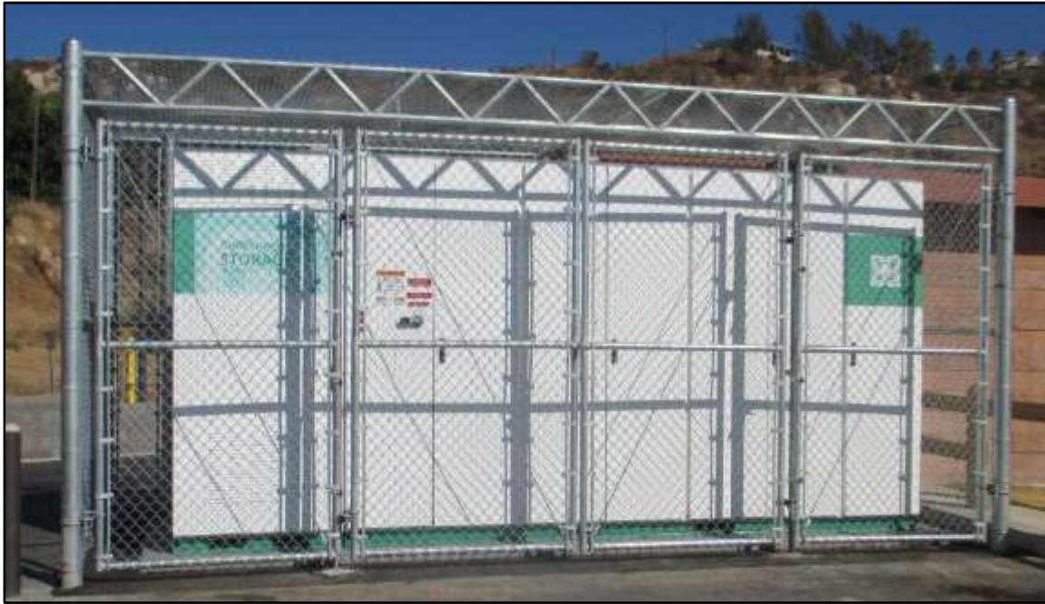
Figure 5: 250kW/500kWh Battery Energy Storage System
