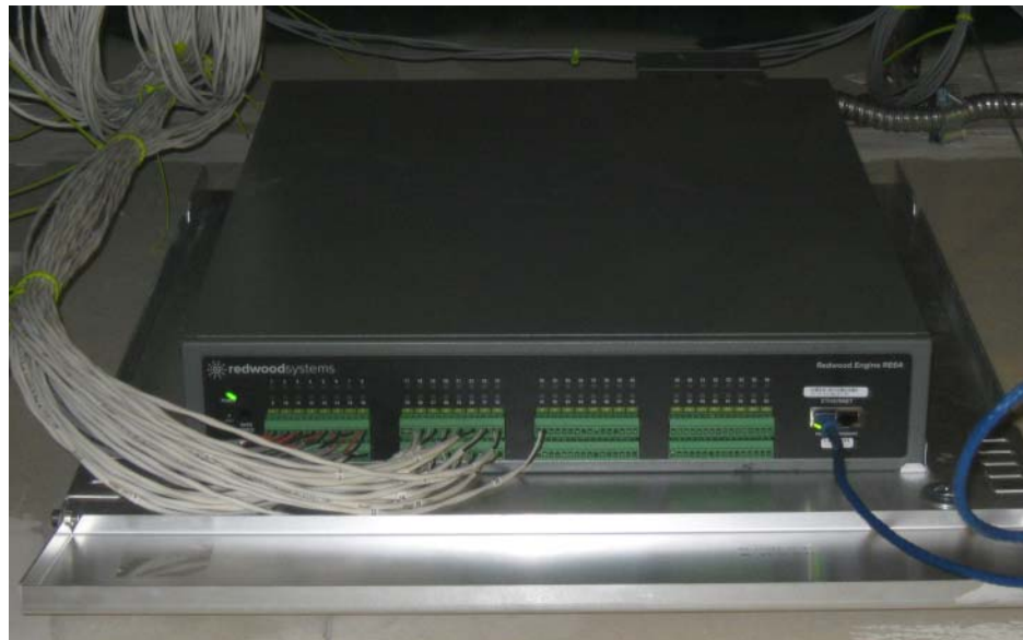
FIGURE 5. REDWOOD SYSTEMS ENGINE FOR CONTROLLING LED LIGHTS
