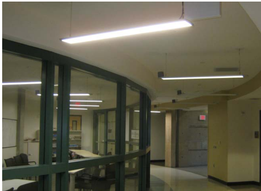
FIGURE 4. CURVED CORRIDOR AND TEACHING LAB LIGHTING
