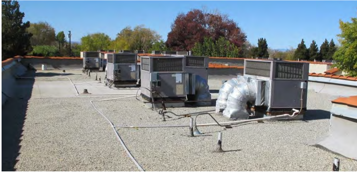
Figure 4: Rooftop Packaged HVAC Units on Building 1
