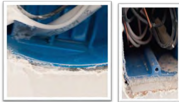
Figure 48: Aerosol Space-Sealing Test for Air Change Rate
