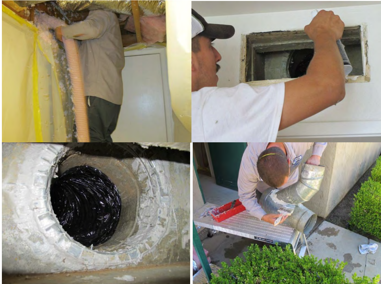
Figure 41: Retrofits to Achieve High-Performance Ducts
