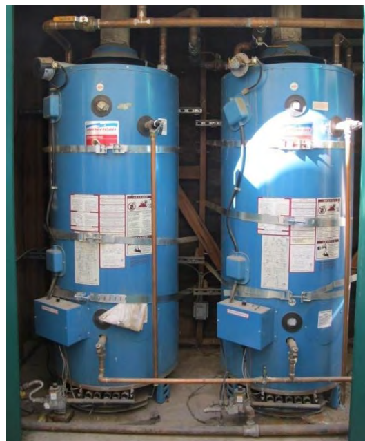
Figure 5: Domestic Hot Water Tanks
