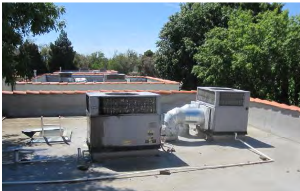
Figure 29: Air Conditioning Units on a Duplex Unit
