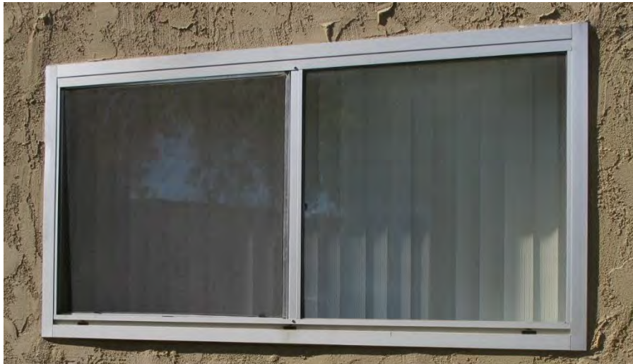
Figure 9: Double-Pane Windows with Metal Frames
