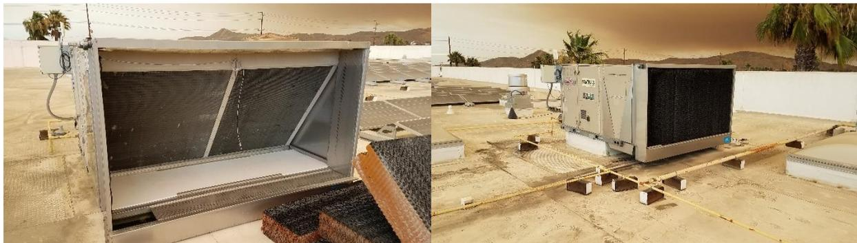
**FIGURE 3: CONDENSER AIR PRE-COOLER INSTALLED ON 10-TON RTUs, (LEFT), SLANTED CONDENSER COIL, (RIGHT), “V” SHAPED CONDENSER COIL.**
