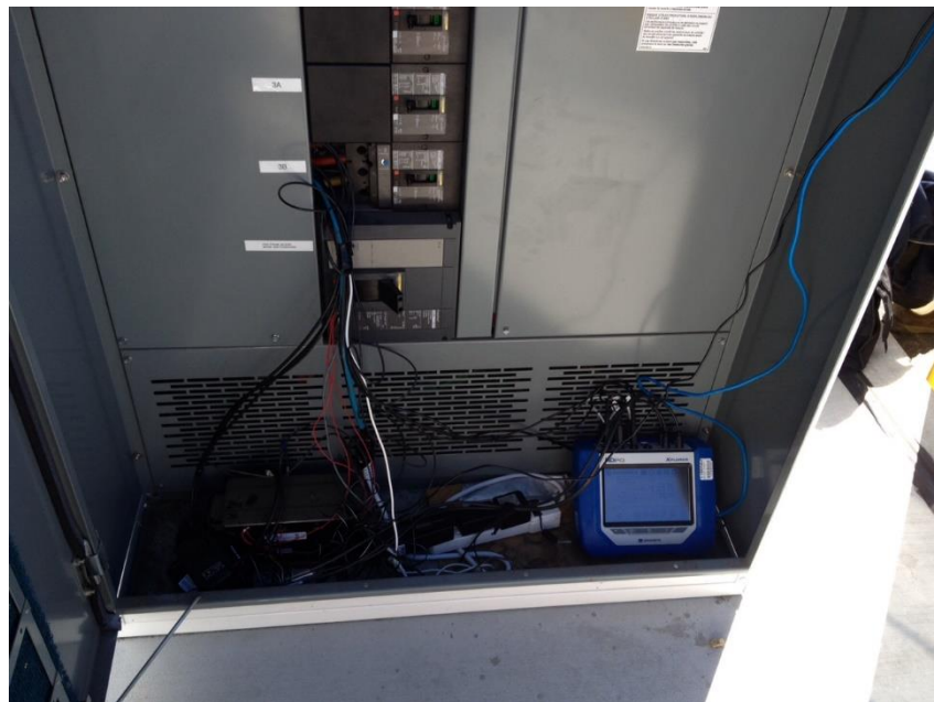
FIGURE 3. CUSTOMER 3 PQ MONITORING INSTALLATION
