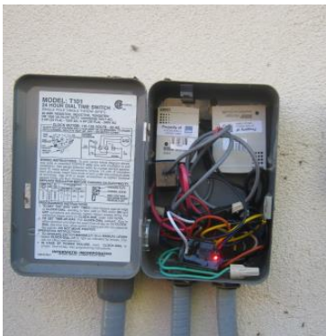
FIGURE 8. CURRENT TRANSDUCER AND HOBO LOGGER IN TIMER BOX
