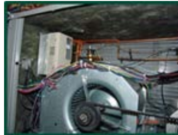
Figure 1: 5-TON RTU fitted with: VFD Controller (left) and ADR Controller (right)
